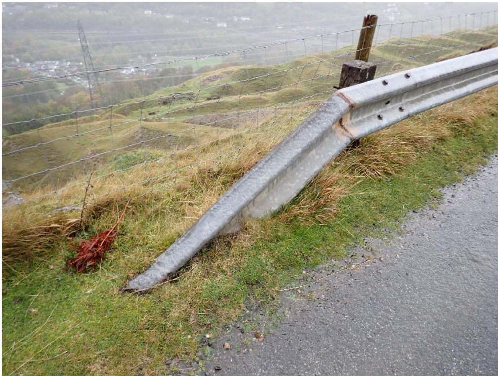
Plate 5: Chainage 64m Start of VRS
